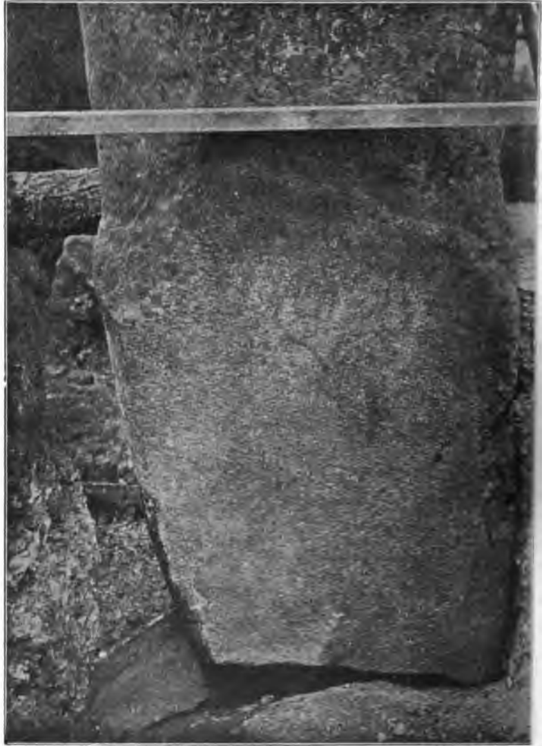
FIG. 8.—The original tooling of the stone protected from the action of the weather.
